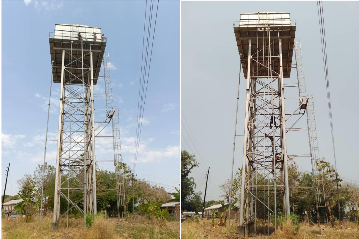
Photos 8: Riser pipes before and after connections to the tank
